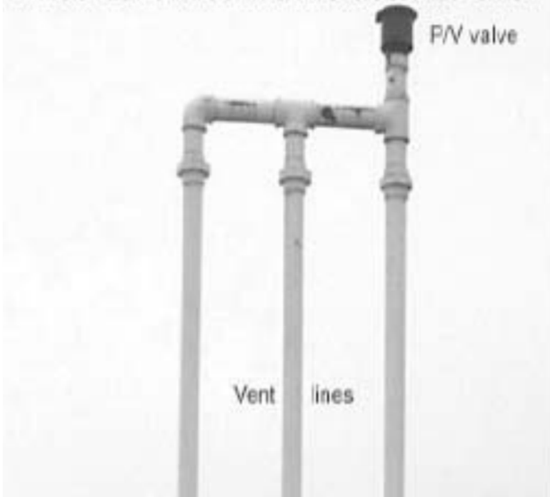
Three vent lines manifolded into one.
